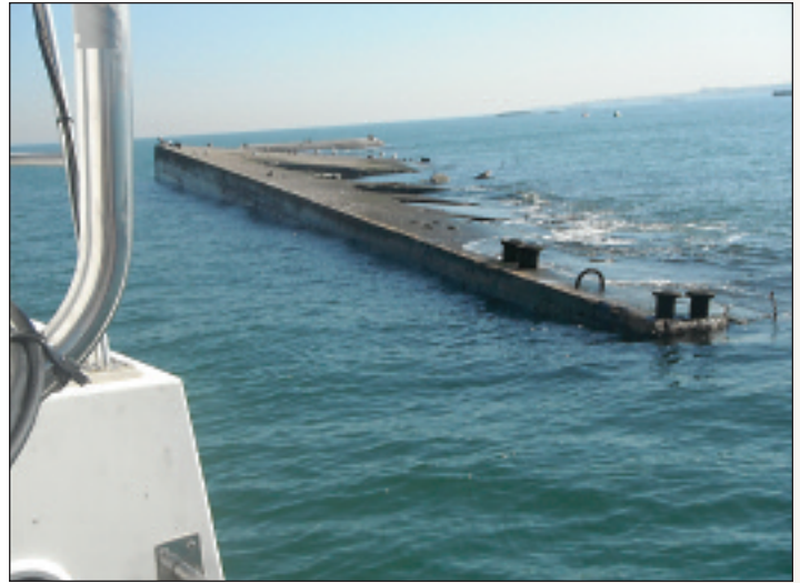
Navigating close to nearly submerged caissons at low water. These caissons are the large AX type, which are 200 feet long, 60 feet wide and 60 feet high. The boat is about 20 feet off the caisson. Only the extremely calm conditions allowed the boat to be this close.
