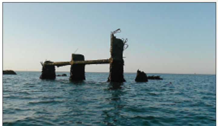
Some of the dangers that remained submerged at high tide but became exposed at low water. The vertical concrete structures and extruding rebar constituted a very real danger for the survey boat.
